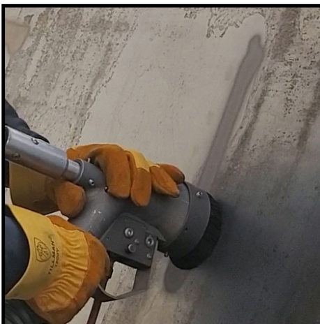
Work head blasting pattern
