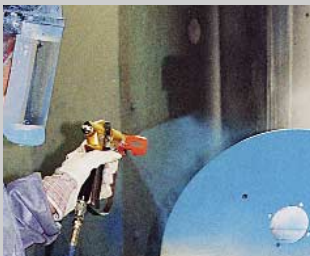
Coating metal surfaces
