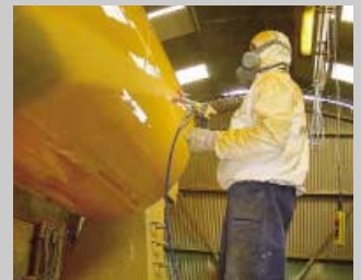
Tank coating in Belgium
