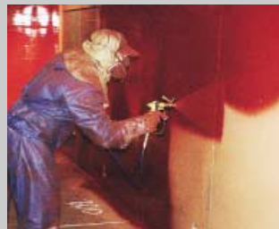
Coating railcars in Poland
